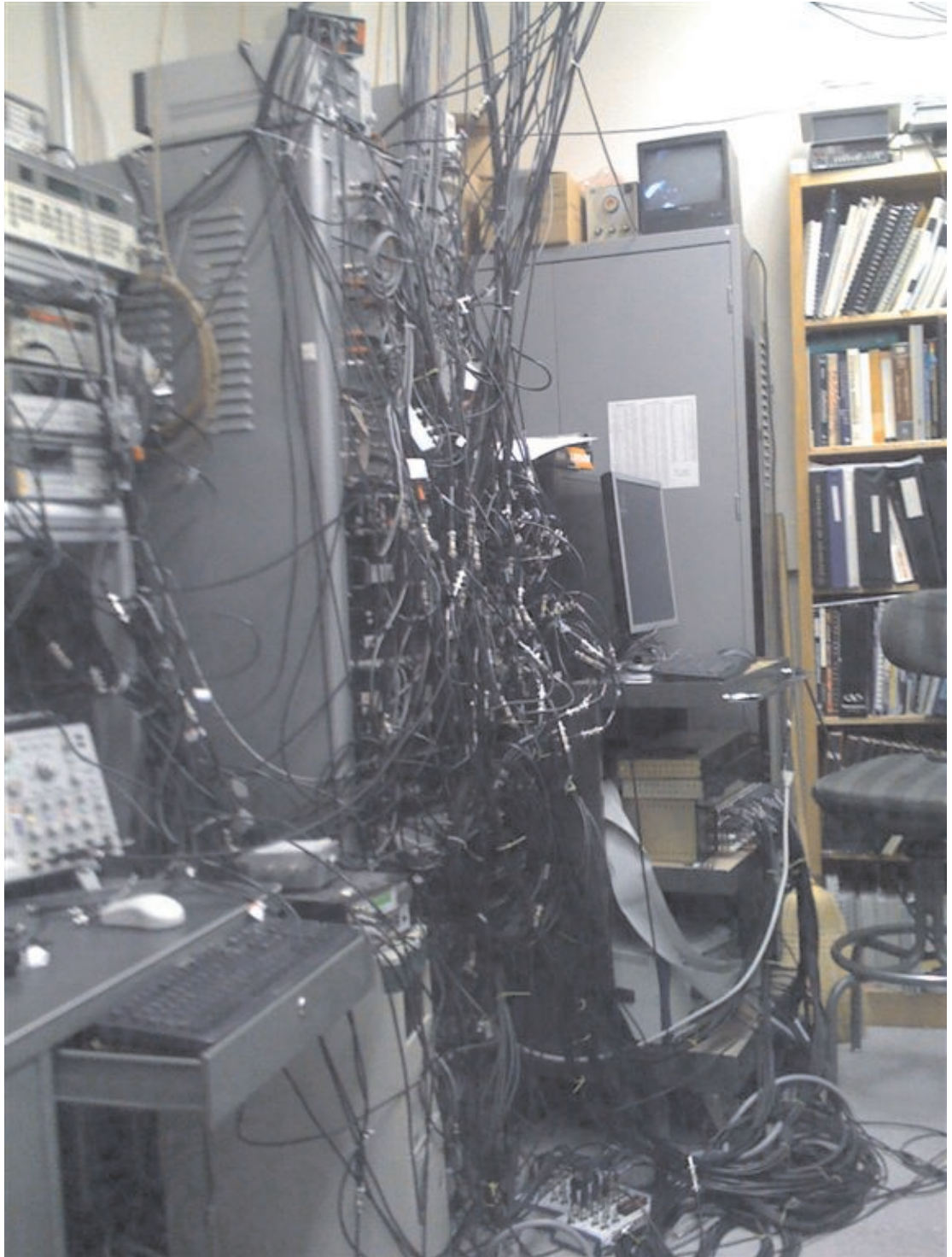
Figure 3.2: A picture of our computer control setup while we were in the middle of switching to our new setup. Switching to a newer setup was a daunting task but thorough preparation resulted in less than one week of downtime.
